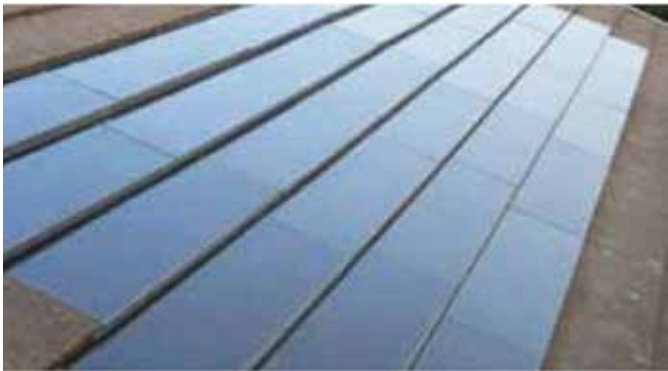
Solar slates integrated into a tiled roof can be virtually indistinguishable when views from the street.
