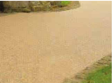
Resin bonded footpath /crushed stone
