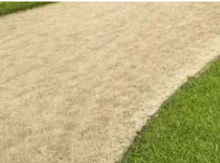
Exposed gravel footpath
