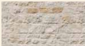
Rough rubble stonework Light cream / grey limestone
