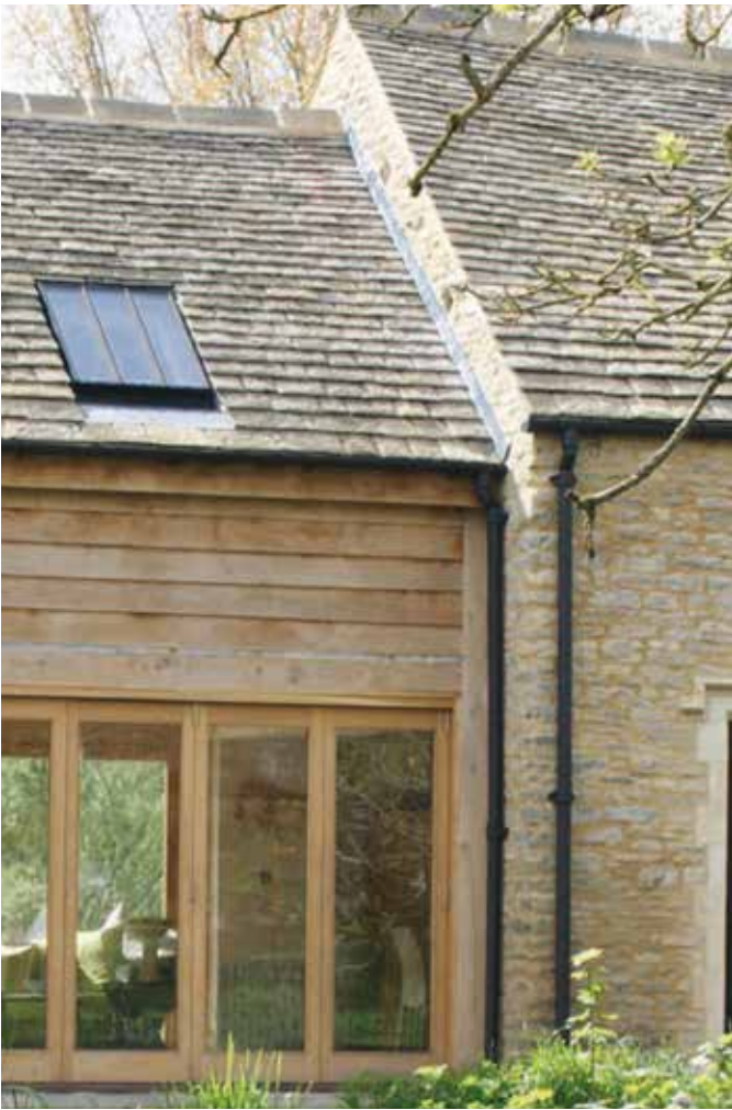
Rubble stone, timber and large glazed areas
