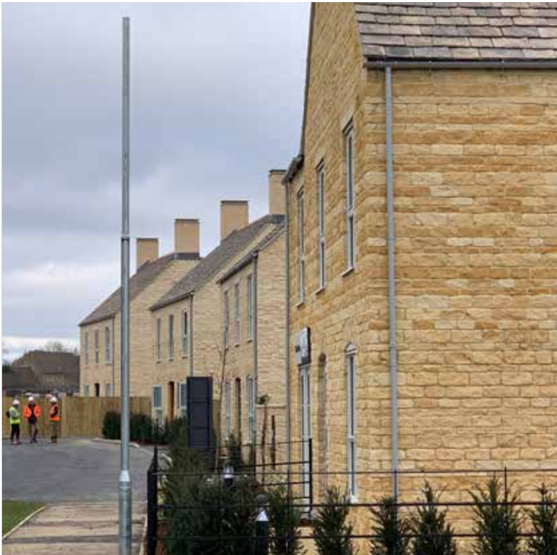
Phase 1 under construction
