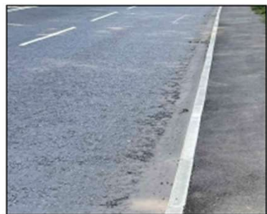
Hot Rolled Asphalt for Carriageway
