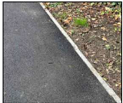
Asphalt Concrete for Footway
