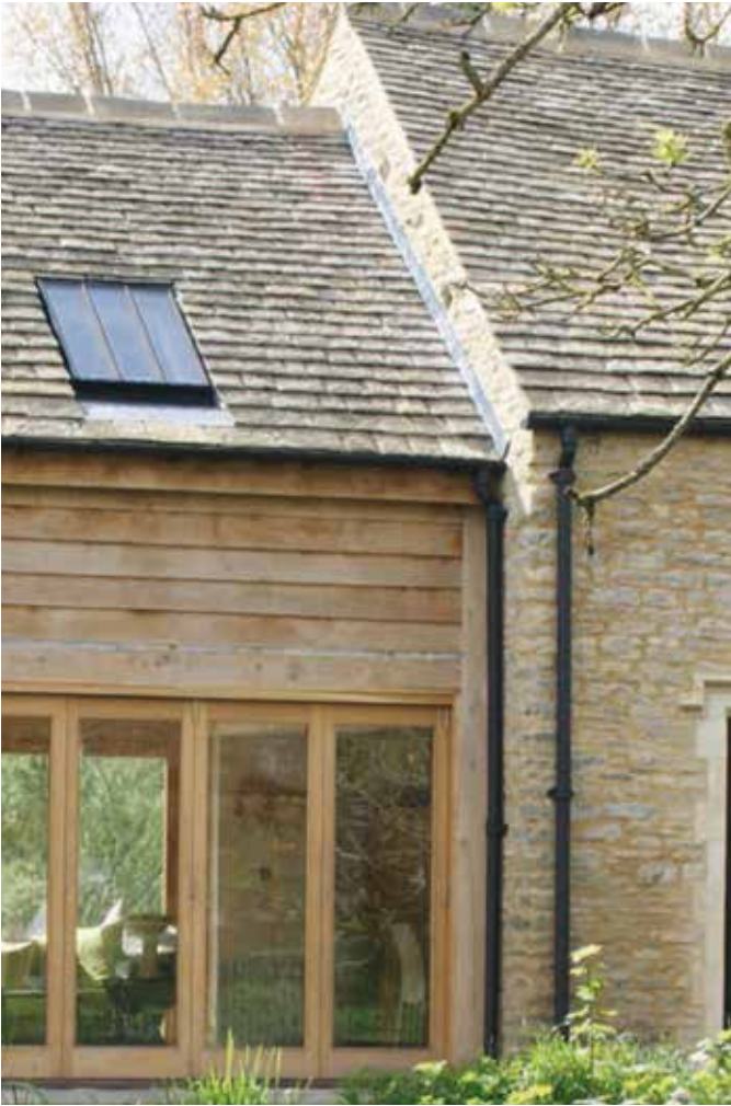
Rubble stone, timber and large glazed areas
