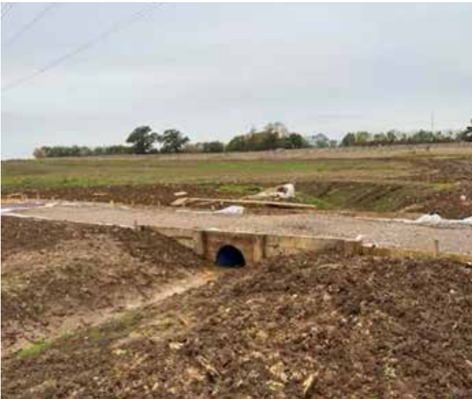
Path over culvert
