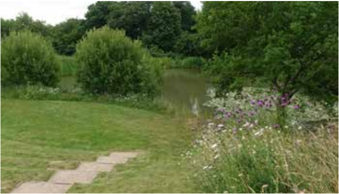
Landscaped attenuation basin
