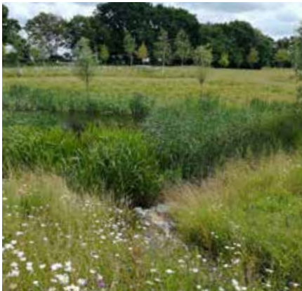
Planted attenuation basin
