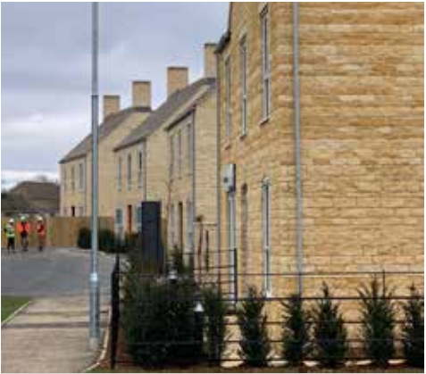
Phase 1 under construction
