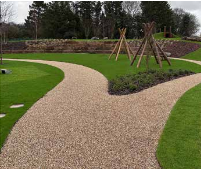
Gravel dressed path with hot bitumen emulsion tack coat installed in Phase 2B
