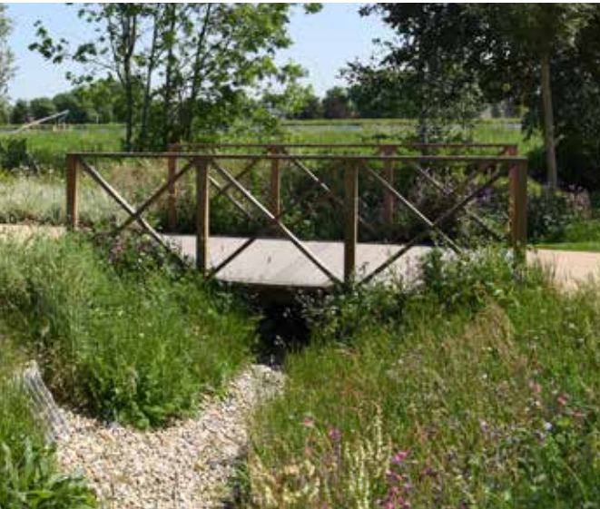
Hardwood timber bridge
